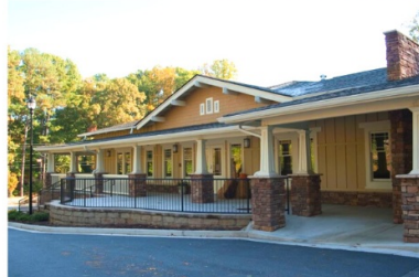
Wolfe Adult Community Center - Bathroom Addition
